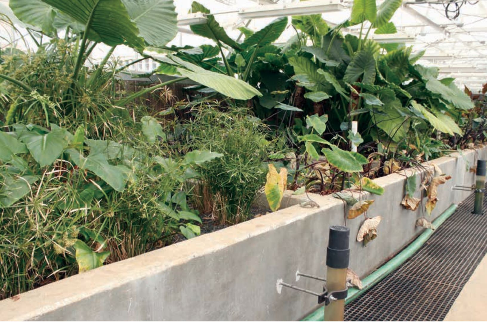
A replicated tidal-flow wetland like this one at Furman University could help UGA save money on wastewater treatment. Photo: Environmental Practicum
